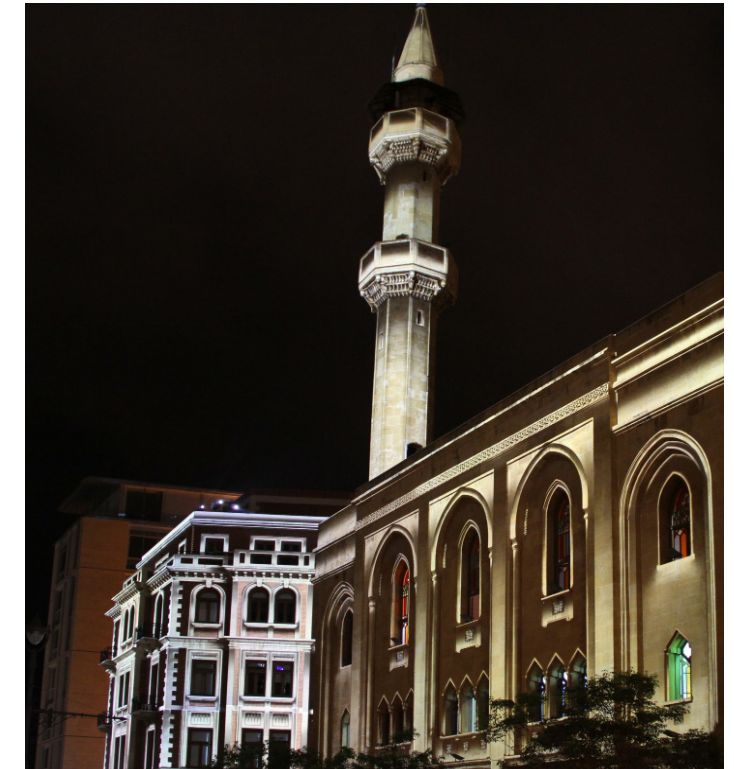
Lighting Beirut Architecture_Lebanon_2011
