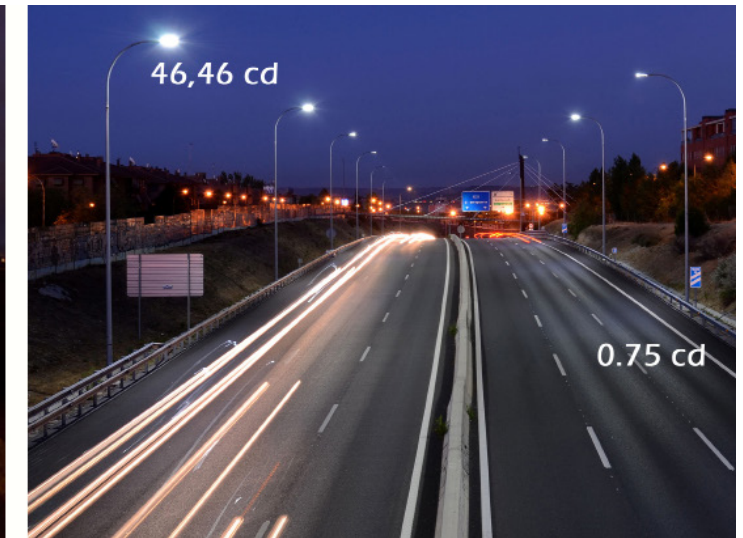
2. Luminance intensity: with cut off light system
